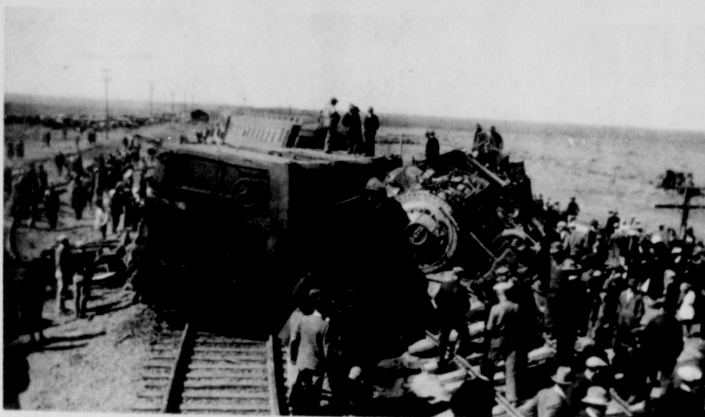
WRECK IN 1926--The train wreck at Posey on Feb. 22, 1926 is remembered as being one of the worst around Slaton. H. T. Shelby, engineer, was killed in the accident. Crowds came from miles to see the massive steam engine that derailed, turned over and plowed through the track and the ground. (Courtesy of Arthur Demas)
