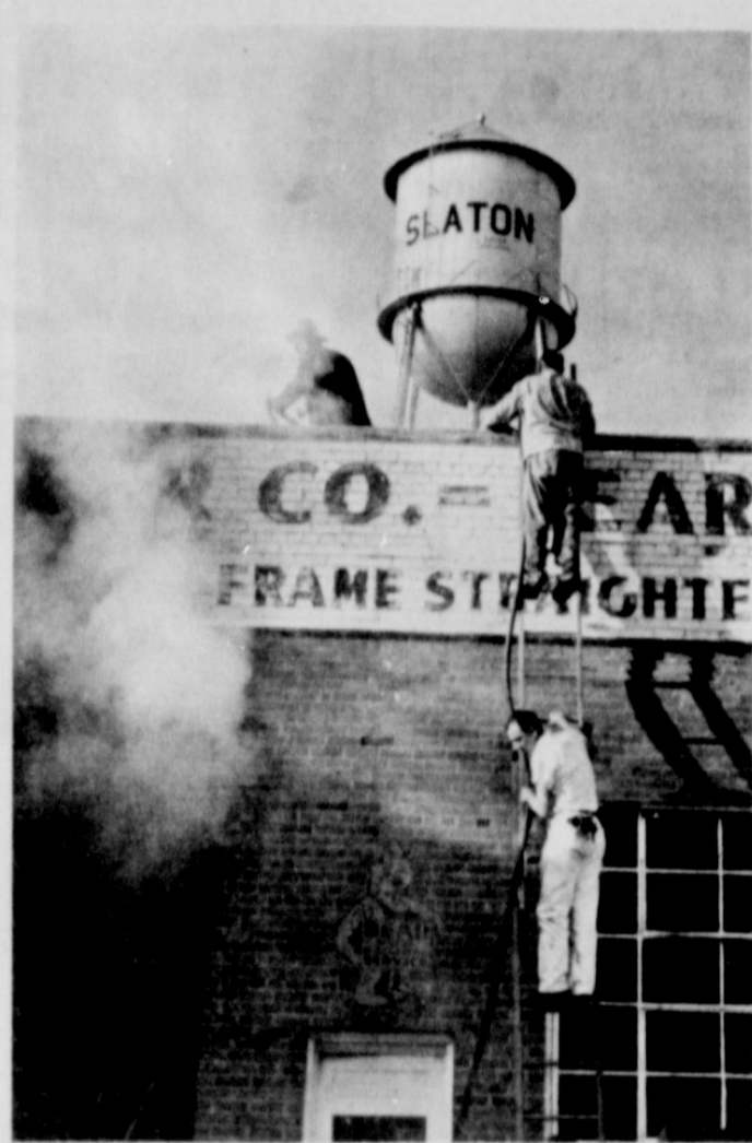
HEAVY DAMAGE--Damage soaring into the thousands of dollars was sustained by the service wing of Smith Ford Friday afternoon. Members of the Slaton volunteer fire department responded to the alarm and extinguished the blaze. One employee suffered minor burns to his hands.
