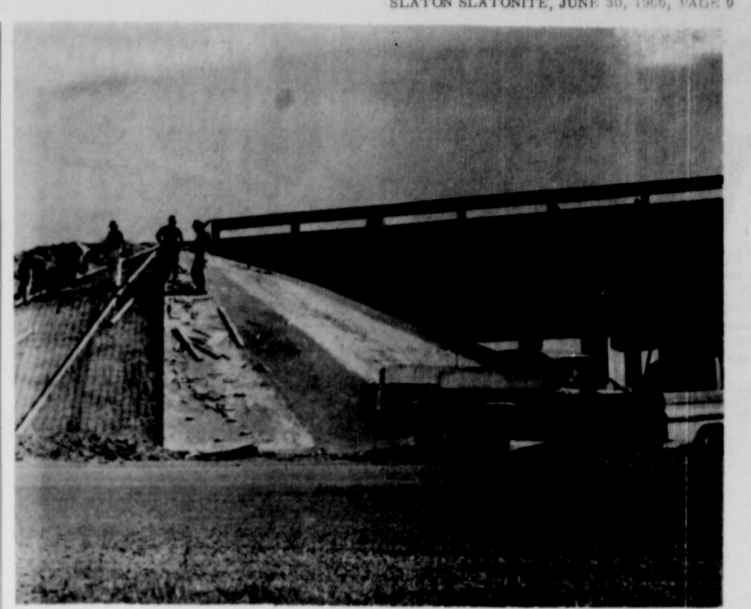
WORK NEARING COMPLETION ON FM 400 - US 84 BY-PASS (SLATONITE PHOTO)
