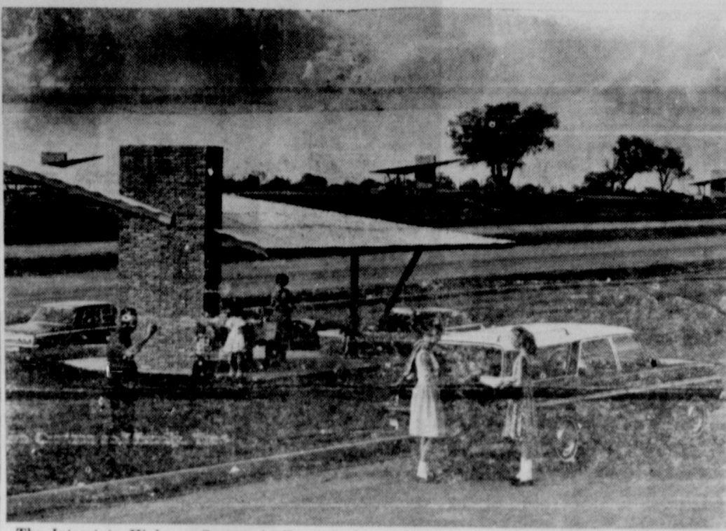
The Interstate Highway System in Texas is being blessed with large, elaborate Safety Rest Areas for the safety and convenience of Texas travelers. Motorists can now relax and refresh themselves in the first of these rest areas (roadside parks) designed and built on the Interstate Highway System in Texas. This new rest area contains eight arbors equipped with fire places for family cooking, incinerators, fire wood, and big spacious tables and benches for picnicking. The "park" lies on a small knoll ten miles east of San Antonio on Interstate Highway 10 and was formally dedicated May 29.
