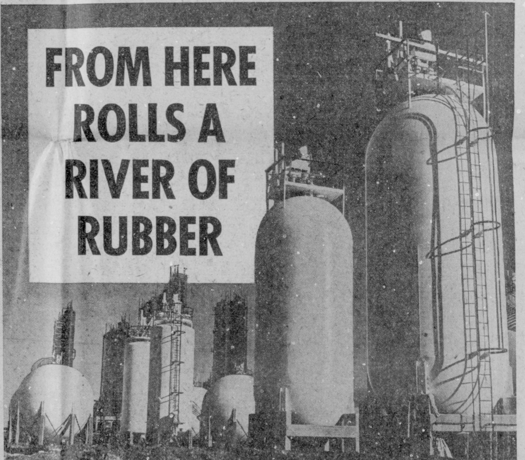
These odd-shaped storage tanks are part of the new plant operated by Sinclair Rubber Inc. for the Government.
