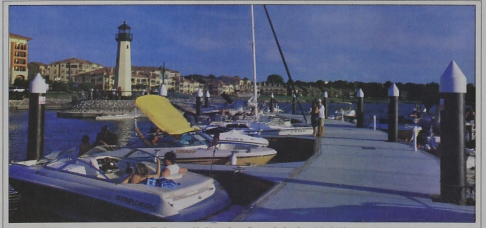
New docks recently constructed at The Harbor provide 41 new boat slips, replacing the original 11 boat slips damaged last year by storms. The new docks also provide room for eight to 10 additional side-ties along the walkways, according to a City of Rockwall news release. The Rockwall City Council authorized construction in late 2009. Photo courtesy City of Rockwall/Rockwall County News
