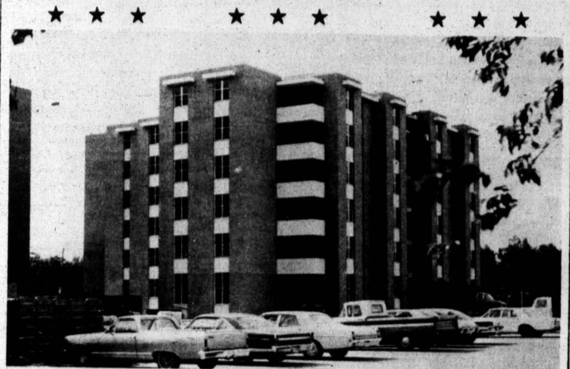
HIGH-RISE — This modern building is one of two new high-rise dormitories at West Texas State that are scheduled to be ready for occupancy by the fall semester. (WTSU Photo)
