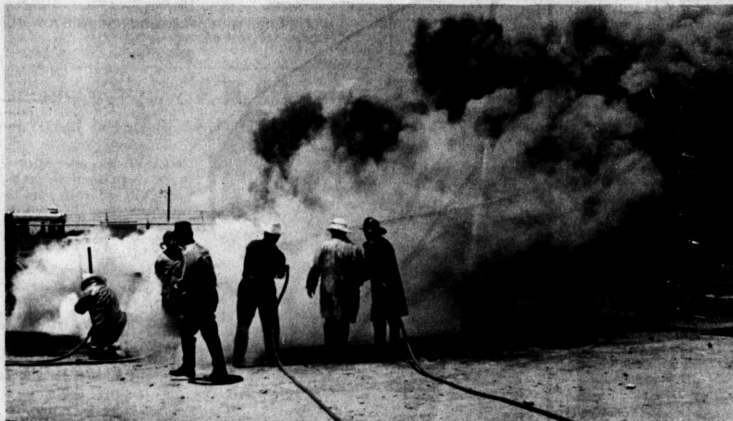
MUCH SMOKE — Billows of black smoke covered the west side of town Tuesday at 2 p. m. indicating a larger fire than really existed. A stack of orange-burg pipe at Jim's Plumbing at 803 S. Texas was evidently ignited by sparks from a trash fire in a nearby underground incinerator. Estimated loss in pipe and other equipment is $600.
