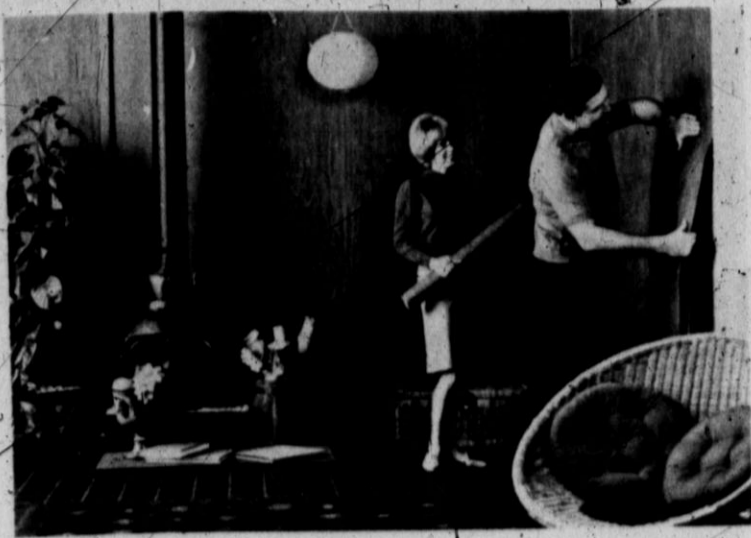
PAINLESS WAY TO PANEL — Rich woodgrain patterns in heavy gauge embossed vinyl go on easily. As backing paper is pulled away, the self-adhesive vinyl is smoothed on the wall to provide a paneled room setting.
