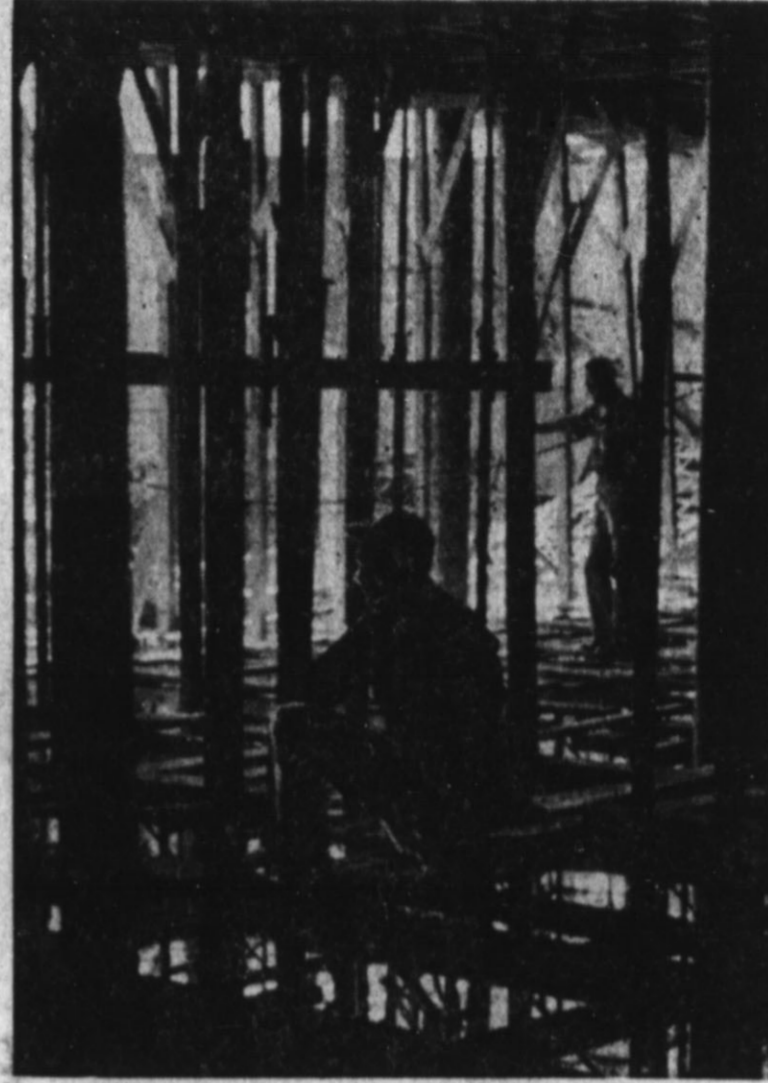
MAZE OF BRACES —Contractor Robert Moxley, background, surveyed damage resulting from the collapse of a section of roof on a million-gallon water reservoir on Ave. C. City Manager Monroe Moore, silhouetted among a maze of braces beneath a segment previously poured, watched workmen putting in additional reinforcements before starting work on another part of the roof. (Staff Photo)
