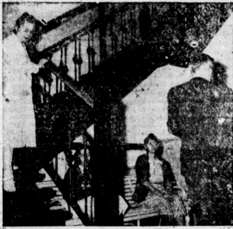
IRON STAIRS IN ABILENE HOSPITAL —This ancient iron stairway at the Abilene State Hospital has caused many falls—not only by the epileptic patients in the hospital, but by the nurses as well. Several patients in the last dozen years have fallen on these stairs and been killed. Injuries occur nearly every week. Notice how cautiously the nurse in the picture is moving from step to step. Abilene State Hospital was one of the several hospitals at which newspapermen of the state recently inspected conditions.
