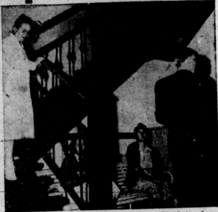
IRON STAIRS IN ABILENE HOSPITAL — This ancient iron stairway at the Abilene State Hospital has caused many falls — not only by the epileptic patients in the hospital, but by the nurses as well. Several patients in the last dozen years have fallen on those stairs and been killed. Injuries occur nearly every week. Notice how cautiously the nurse in the picture is moving from step to step. Abilene State Hospital was one of the several hospitals at which newspapermen of the state recently inspected conditions.
