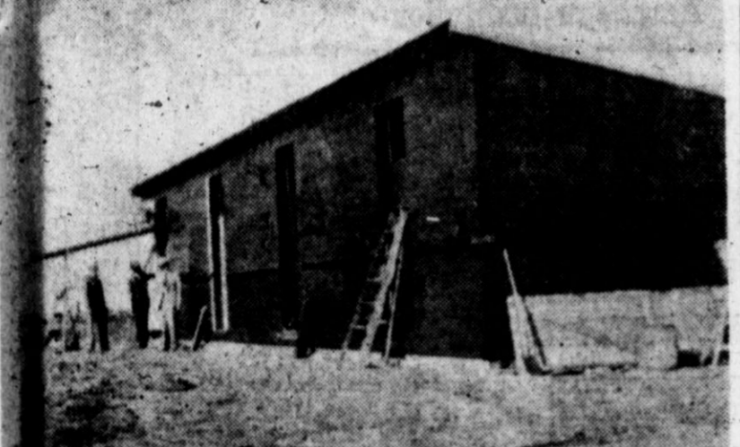
LAWFORD FARM GRANARY —Henry Crawford has one of the average on-bin storage type granaries on his farm east of town. Faust Collier, local PMA administrator, Wes Bradley and District Administrator Dale Carter of Amarillo are examining the building. Photo courtesy Times.
