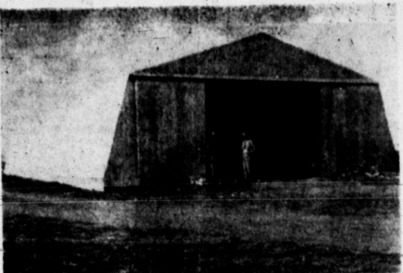
GALLAGHER BARN —This new storage barn on the John Gallagher farm east of town was built recently under the PMA program. Faust Collier and Wes Bradley are standing in the door. Many 30,000-bushel granaries have been built in the county. Courtesy Times.
