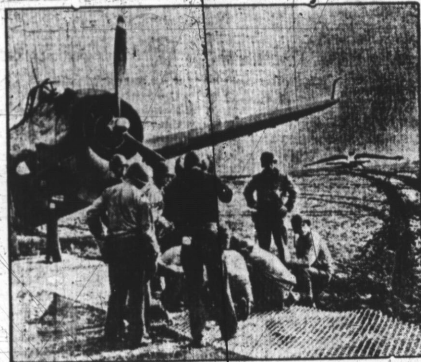
METAL MATS FOR DESERT TAKEOFF—When Anglo-American forces occupied North Africa, torpedo planes took off in the desert on metal mats like this one, which formed temporary airfields.
