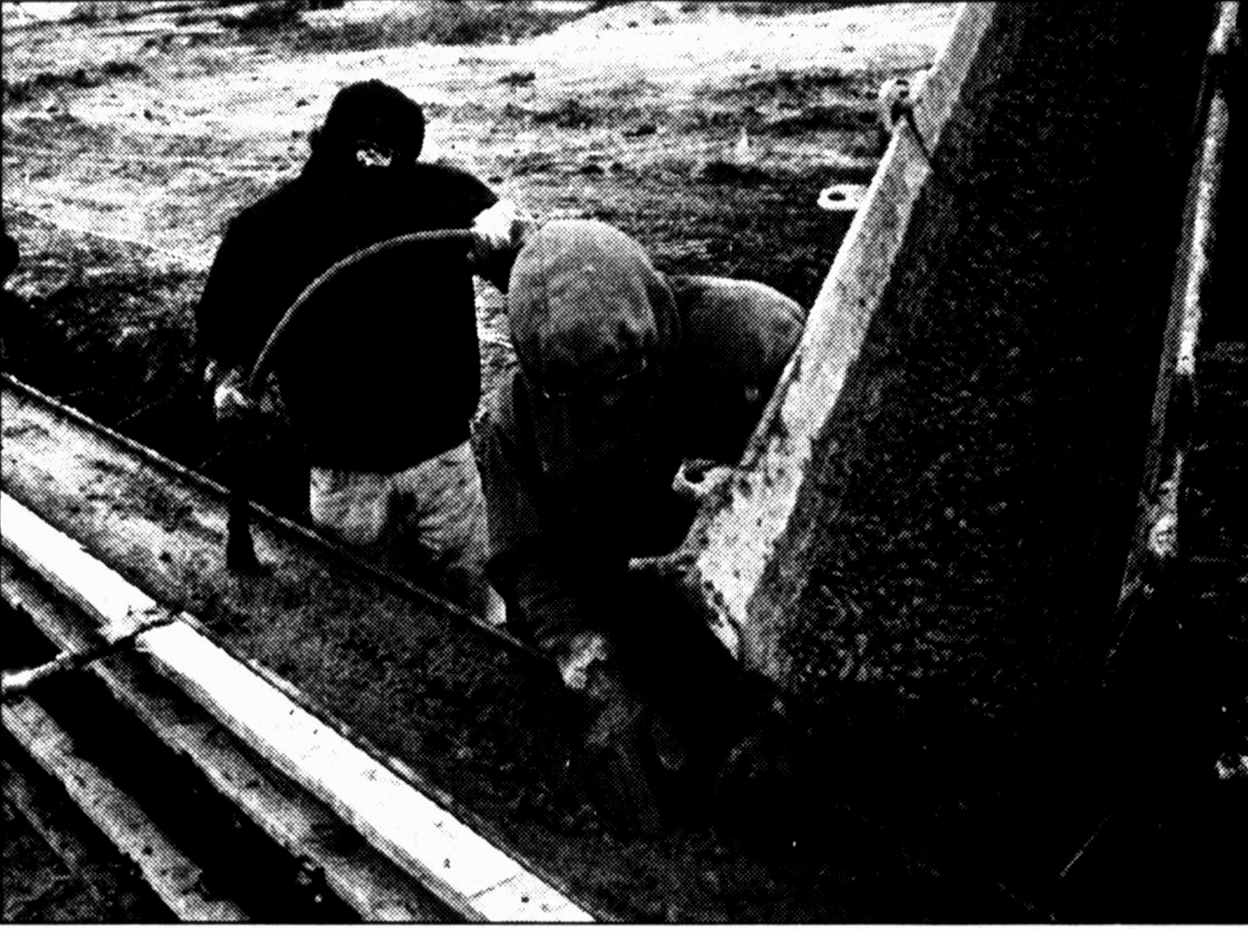
Pouring cement — It was a cold and blustery day to be playing in the wet cement, but concrete workers Janell Cortez, left, and Ron deJongh spent the day Tuesday, doing just that. The construction is part of the foundation to the new Jr. High addition.
