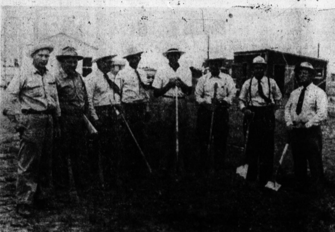
GROUND BREAKING —T. E. Seigler, Jr., president of the REA board, with members of the board and others, officially breaks ground for the new Deaf Smith County REA building now in process of construction on Highway 60 just east of the Hereford city limits. Those present for the Thursday ceremony starting work on the near $100,000 building are from left, Emerson Roland, line foreman; A. R. Ratliff, construct on superintendent; Leo Forrest, REA manager; H. H. Miller of Dawn, secretary of the board; Selgier, Sloan Osborn, vice-president of Friona; Joe Birkenfeld of Nazareth and De wey L. Wright of Dimmitt, members.
