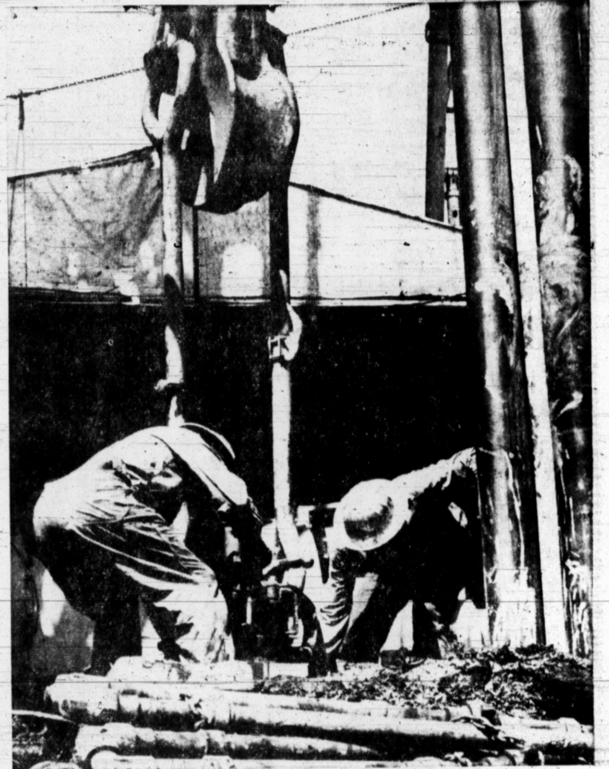
COMING OUT —The derrick man and a roughneck attach the crown block to the top of the drill pipe to pull it out while running the drill-stem test. (Staff Photos)
