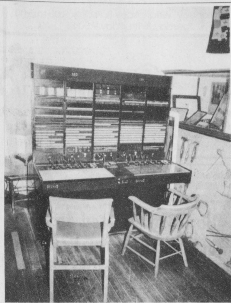
SWITCHBOARD - Bob Myers donated an old switchboard that was used in the Fargo area. Go by the Stationmaster's House Museum and take a step back in time.
