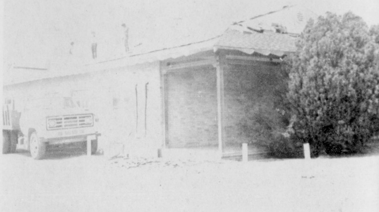
Gruver's Golden Age community center is being repaired with the help of donations including a recent grant from Pioneer Hi-Bred International, Inc.
