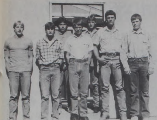
THE ADVANCED WOODSHOP students of Muenster High School are constructing a 10x10 storage building as a class project. Students learn the principles of residential construction. Pictured are, 1 to r, front - Russell Simmons, Alan Hudspeth, Rodney Knabe, Travis Klement, Justin Ashley; back - Weldon Hermes and Mark Rigby.
