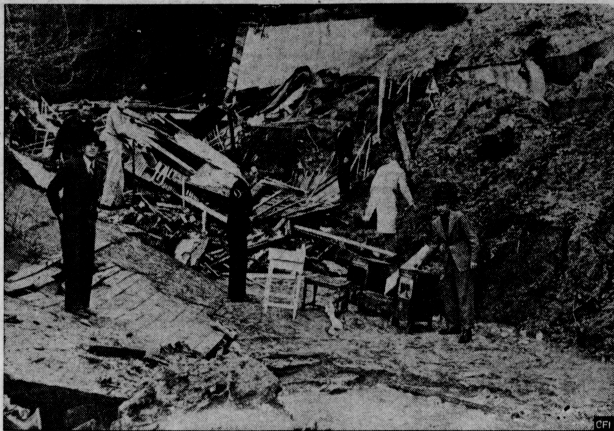
LOS ANGELES, Calif.—This picture shows workmen searching the ruins for the body of Warren A. Atherton who met death when his house collapsed into the street at 2066 Los Encinos Street, Glendale. Flood waters weakened the foundation and sent the house crashing into the street with tons of dirt burying it.
