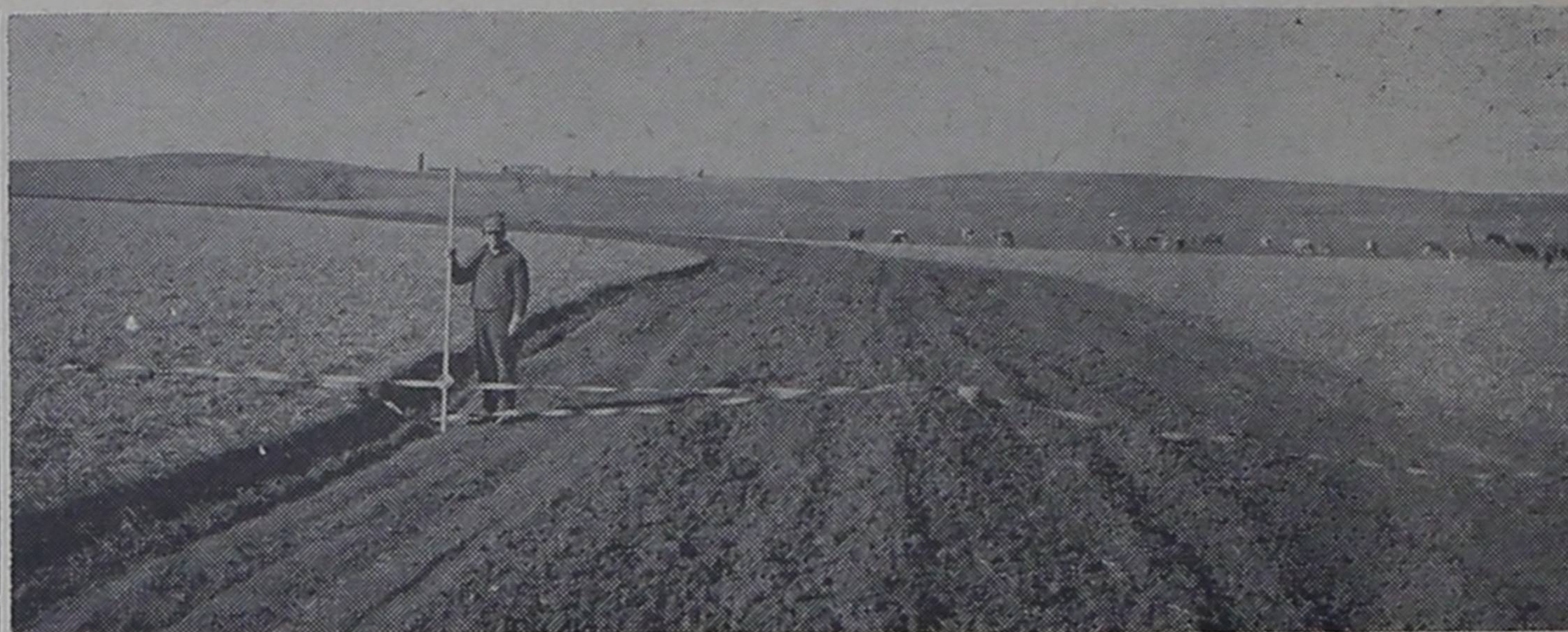
THOMAS SICKING HOLDS A SURVEYING ROD IN THE CHANNEL of one of his plow built terraces to show the depth of water it will carry. A paper tape is stretched over the terrace ridge and channel to show the outline of the soil. Sicking built 3,000 feet of field terraces to protect a sloping field. They were built with a three disc plow and empty onto a Bermuda grass waterway along a natural drain. Soil Conservation Service personnel say that the Muenster area still needs 1,923 miles of terraces to give needed protection to the sloping farmlands. Field terraces can be built with farm equipment or on a contract basis. Cost sharing benefits to assist in the cost of building terrace can be obtained through the Agricultural Conservation Program.
