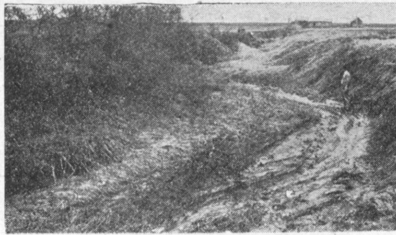
RESULTS OF TERRACING BEFORE OUTLETS WERE SODDED. Terraces without sodded outlets often do more harm than good.
