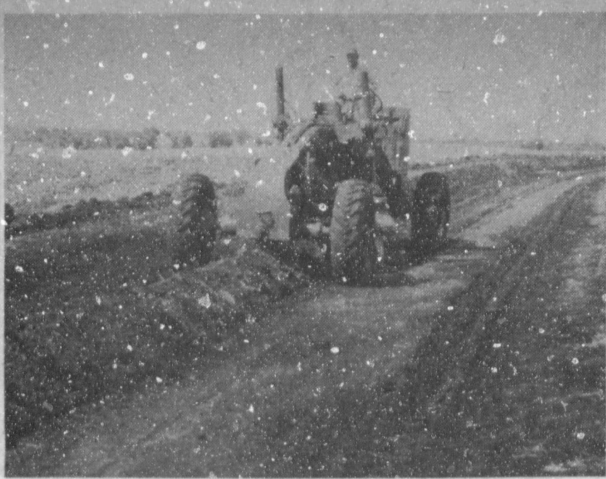
BROAD EASY-TO-FARM CHANNEL TYPE field terrace near Muenster being built by motor grader. The grader is shown making the first half of the final round on the terrace. The terrace has an 8 foot wide flat channel, the terrace ridge is 20 feet wide and 1.4 feet in height from channel bottom. These wide terraces are easy to farm and are well liked by farmers in this area. Over 50 miles of this type terrace were built by Muenster farmers last year. Ray Otto is operating the motor grader.
