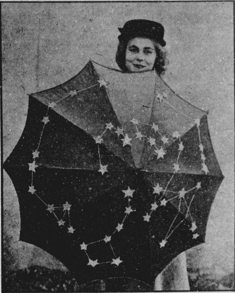
BUMBER-SHOOTING STARS —Clouds may hide the skies, but stars will still twinkle for the user of this umbrella. A rainy-day brightener from West Berlin, Germany, the umbrella has tiny bulbs that light under each star when the user presses a switch. Power is supplied by a battery in the handle.
