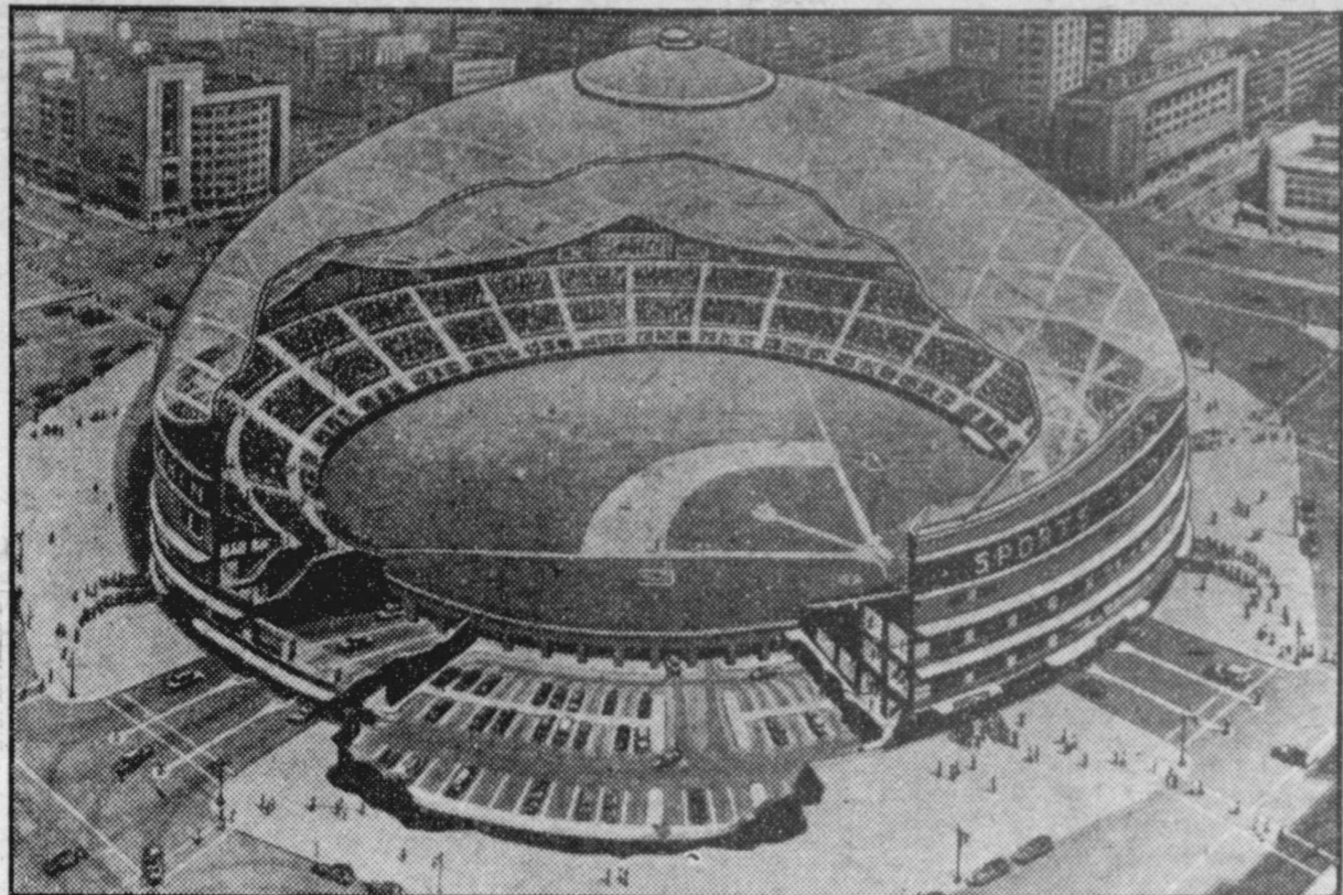
THERE'D BE NO RAINCHECKS —The future home games of the Brooklyn Dodgers may be played under a huge plastic dome, if current plans are followed through. Architect Buckminster Fuller claims the huge, cup-shaped roof over the baseball field would be 300 feet high and 750 feet in diameter. The air-conditioned, all-weather sports center would have a seating capacity of more than 55,000, as compared to 32,000 for Ebbets Field. Artist Frank Tinsley envisions a cut-away view of the finished stadium, above. This artist's conception of the huge sports facility is from July issue of Mechanix Illustrated .
