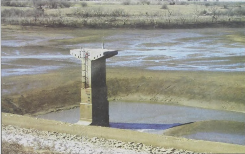
The Muenster Lake spillway tower once more stands tall out in the "water" now that the Lake's contents have been drained.
