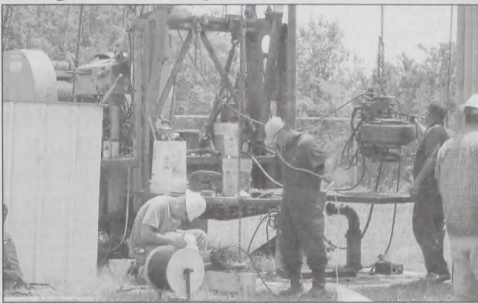
Muenster City Well No. 7 was pulled Tuesday by Biffle Water Well after a submerged motor quit working. Approximately 600 feet of pipe was removed to get to the problem. The motor was replaced and the well was pumping late Tuesday night. Janie Hartman photo
