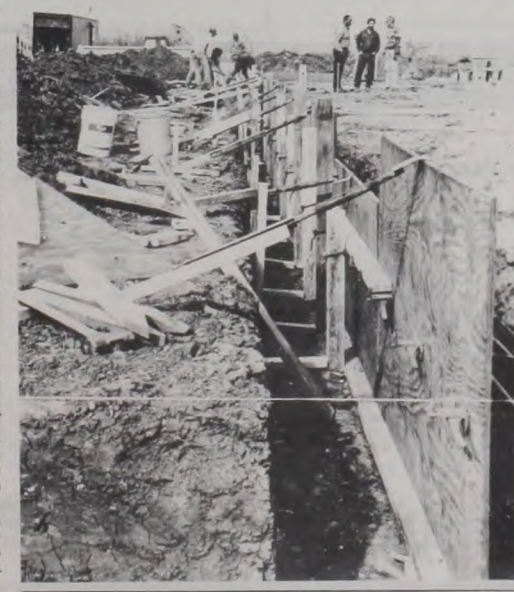
Concrete work by the Dangelmayr and Barnhill Companies continues in preparation of pouring the beam foundation for the new Muenster High School. Above Erik Walterscheid and Jeremy Walterscheid do manual make-ready groundwork.
