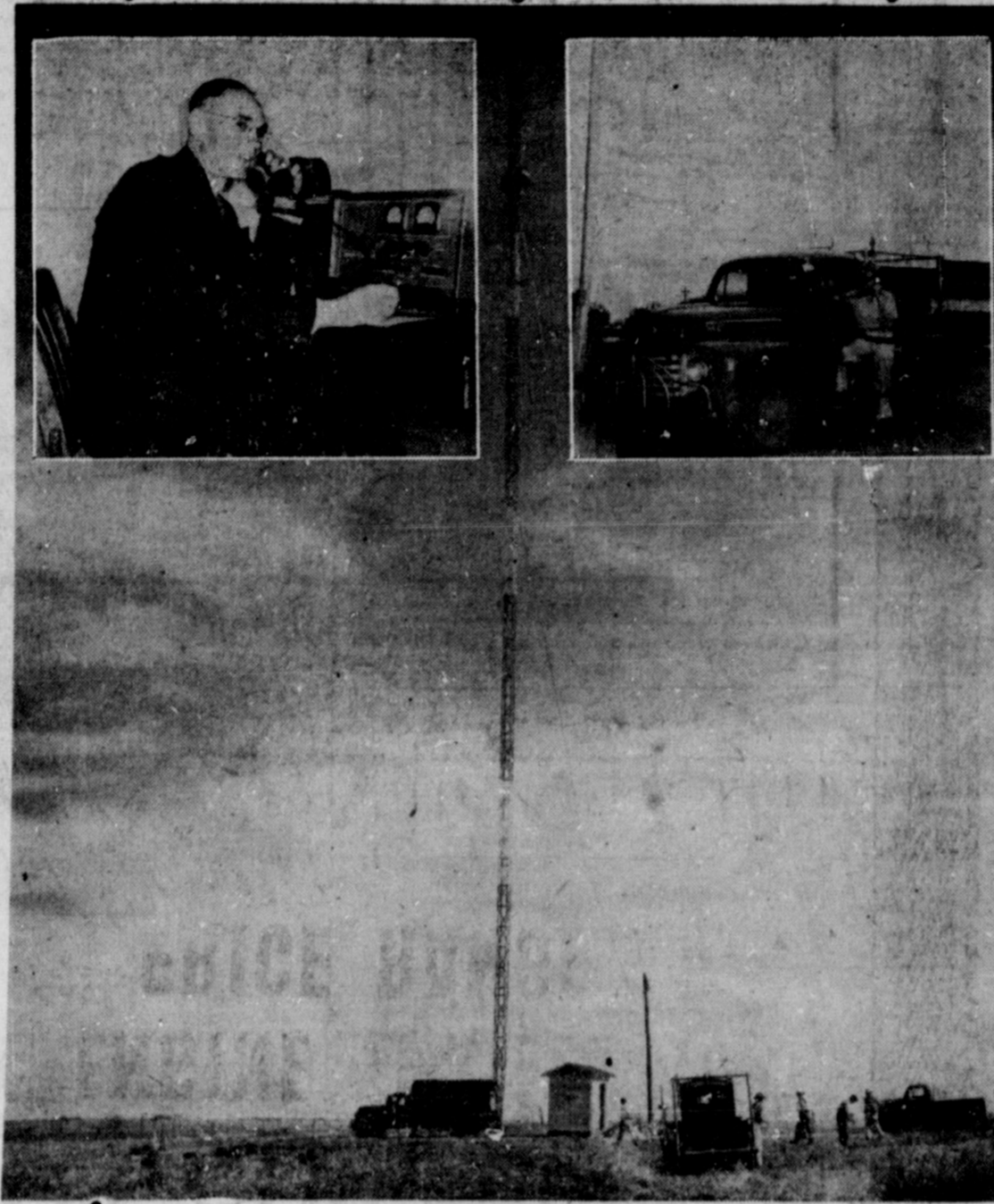
WTU CO.'s NEW TWO-WAY RADIO SYSTEM—"Station KGHQ calling Car J-3, calling Car J-3". That's the call when Carl Hudson, upper left, WTU Co. local manager, Childress, Texas, contacts Bob Adams, WTU Co. Serviceman to give emergency instructions over the new short wave radio system, which went into operation recently.
