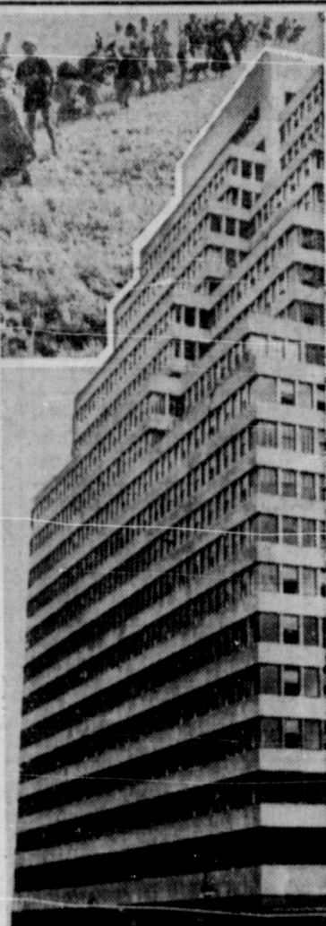
GLASS SKYSCRAPER —Newest tower puncturing New York skyline is shimmering Universal Pictures Bldg., whose 30,000 square feet of glass, according to Libbey-Owens-Ford, projects daylight a record 40 feet into its interior.
