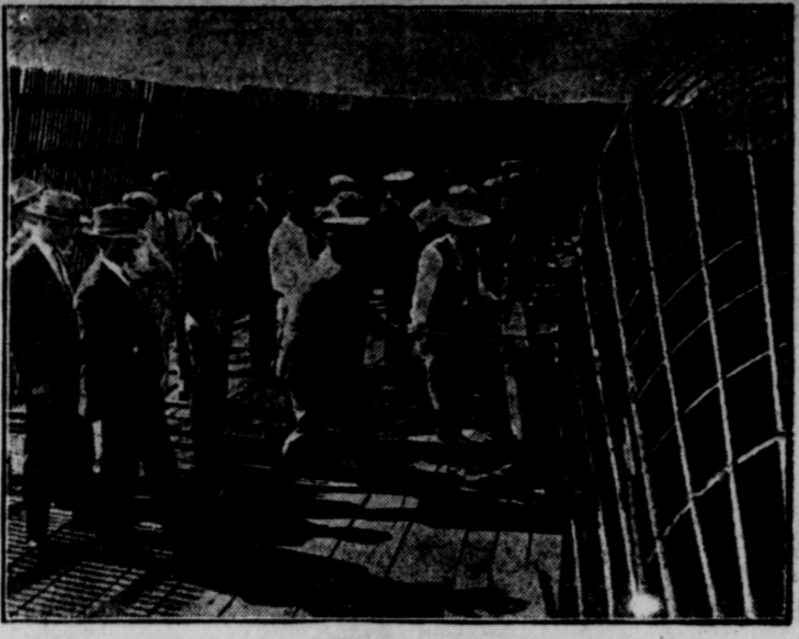
NEW ALL-METAL DIRIGIBLE UNDER CONSTRUCTION AT GLENDALE, CALIFORNIA
