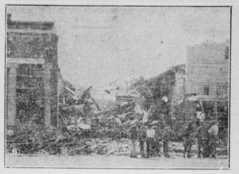
Here is the scene of the downtown gas explosion at Panhandle, Texas, which resulted in injury to four people and $50,000 damage. The blast occurred when W. H. Rogers, grocer, struck a match to look for a gas leak. Rogers, J. I. Raines, Roscoe Vance, Ed Baker, and his son, Esco Baker, were all injured, and three buildings were damaged, one being completely demolished.
