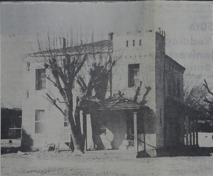
OLD DONLEY COUNTY JAIL* fallen into disrepair and inadequate for holding persons detained by law enforcement officials.
