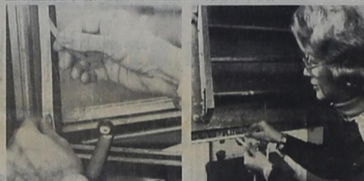
French doors and windows require special weatherstripping which self-adheres to jamb. Foam shape is used to seal attic access. It self-adheres to the attic door.
