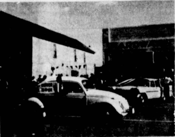
THE TWO STORY building shown above is a landmark believed to have been moved into Hedley from Rowe.
