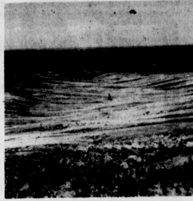
THIS SIX FOOT gully was filled and shaped and then planted to grass, one of the things done every year for soil conservation. Reclamation of eroded land is done through the Great Plains program and this year about 35 acres have been serviced. Soil Conservation Service represents the Donley County Soil and Water Conservation District. For additional information contact Jim Donaho at the SCS office.
