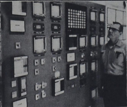
LEFT TO RIGHT: 1. Greenbelt Lake; 2. Greenbelt Water Authority; 3. Operation Supervisor, Frank Drummond demonstrates a new turbidimeter. This instrument measures the turbidity of the raw and finished water each day. Finished water can't exceed 1 turbidity unit. The average turbidity for our water in December was; raw 5.14; treated .289. 4. Plant operator, James Swearingen explains the instrument panel at the water treatment plant. These indicators are frequently monitored for any deviation from normal.
