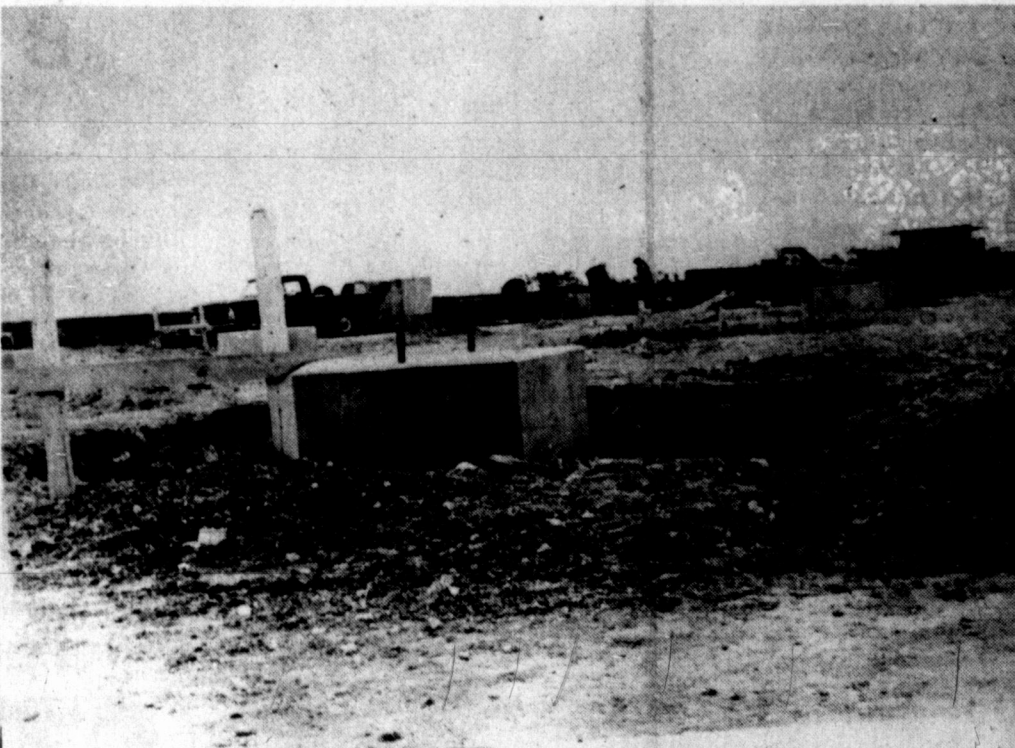
Greenbelt's water systems under construction
