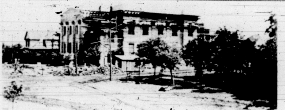
METHODIST CHURCH under construction 1910
