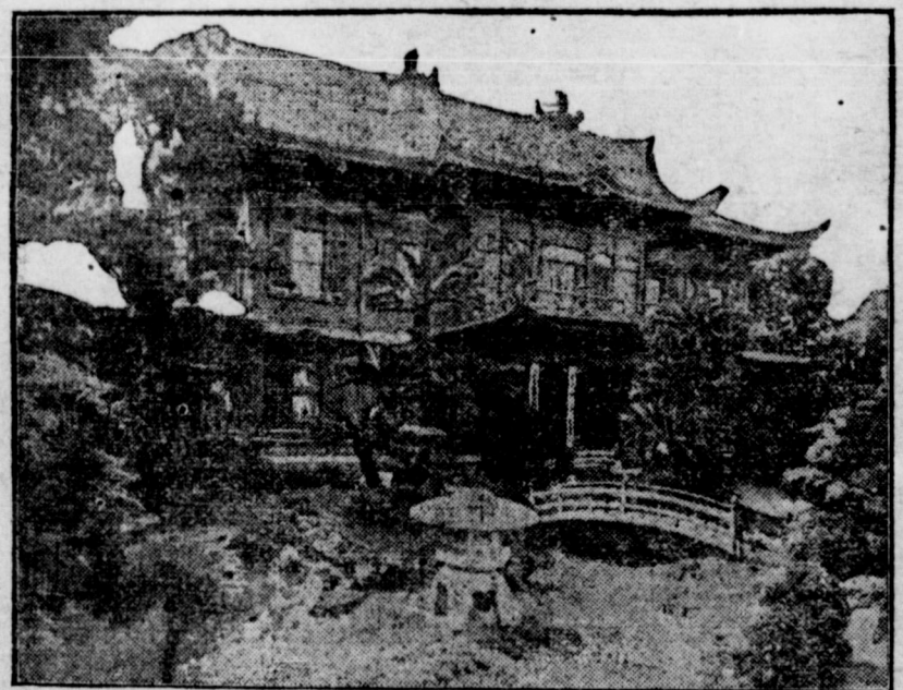
The Roof With the Devil in It. (The Devil Around Corner to the Left Cannot Be Seen.)
