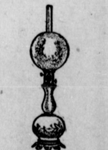
(1800) modification of the Argand lamp by Carcel; oil in base is raised by clock-work pumps.
