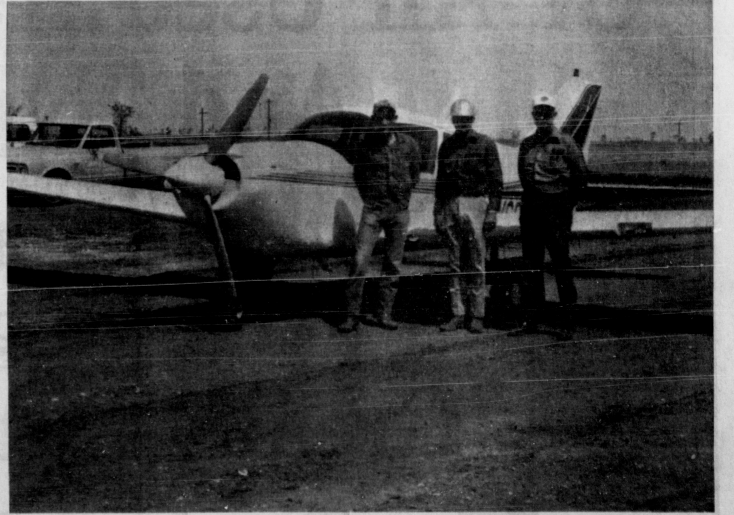
FIRST PLANE LANDS ON HOWARDWICK STRIP—Raymond Newell, right, of Canadian was the first to put his plane down on the new Howardwick air strip which is under construction at this time with most preliminary dirt work completed. Pictured with him at left, Corky Wilson, owner and operator of the lease and Ira Page, contractor. The strip will have a six inch base, lights etc. except for surfacing which is scheduled for next year. Wilson plans to have fueling facilities within the next few days and will also start his hanger and service building which will hold six planes. —Photo by Saye's
