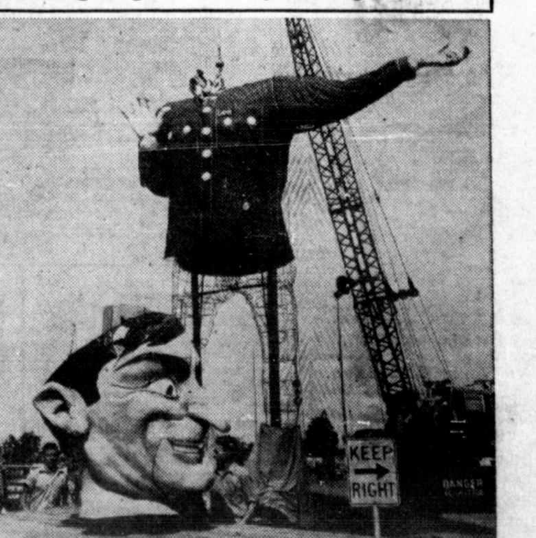
"Big Tex," the towering 52-foot cowboy statue who symbolizes the great State Fair of Texas, is being put together in readiness to welcome some two-and-a-half million visitors to the 1958 exposition, October 4 through 19, in Dallas. It takes a crew of workmen with a 100-foot derrick to put the big boy's head on his shoulders.
