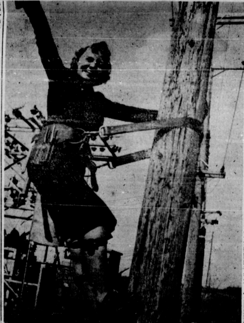
The West Texas Utilities alone had 200 men at work at one time repairing damage wrought by the Panhandle's worst ice and sleet storm. Among volunteers who pleaded for the assignment of "helping out" was a girl, Miss Sarah Smith, WTU cashier at Anson, who said: "I think it's the neighborly thing to do." She proved her willingness by squirming up a 50-foot power line pole.
