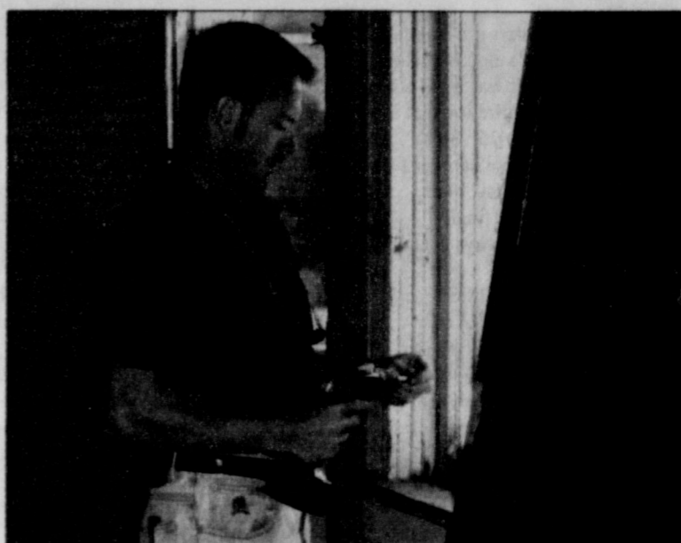
Emmett Longly with Phoenix I installs new hinges on a door in the old Ft. Worth & Denver Railroad Depot.
