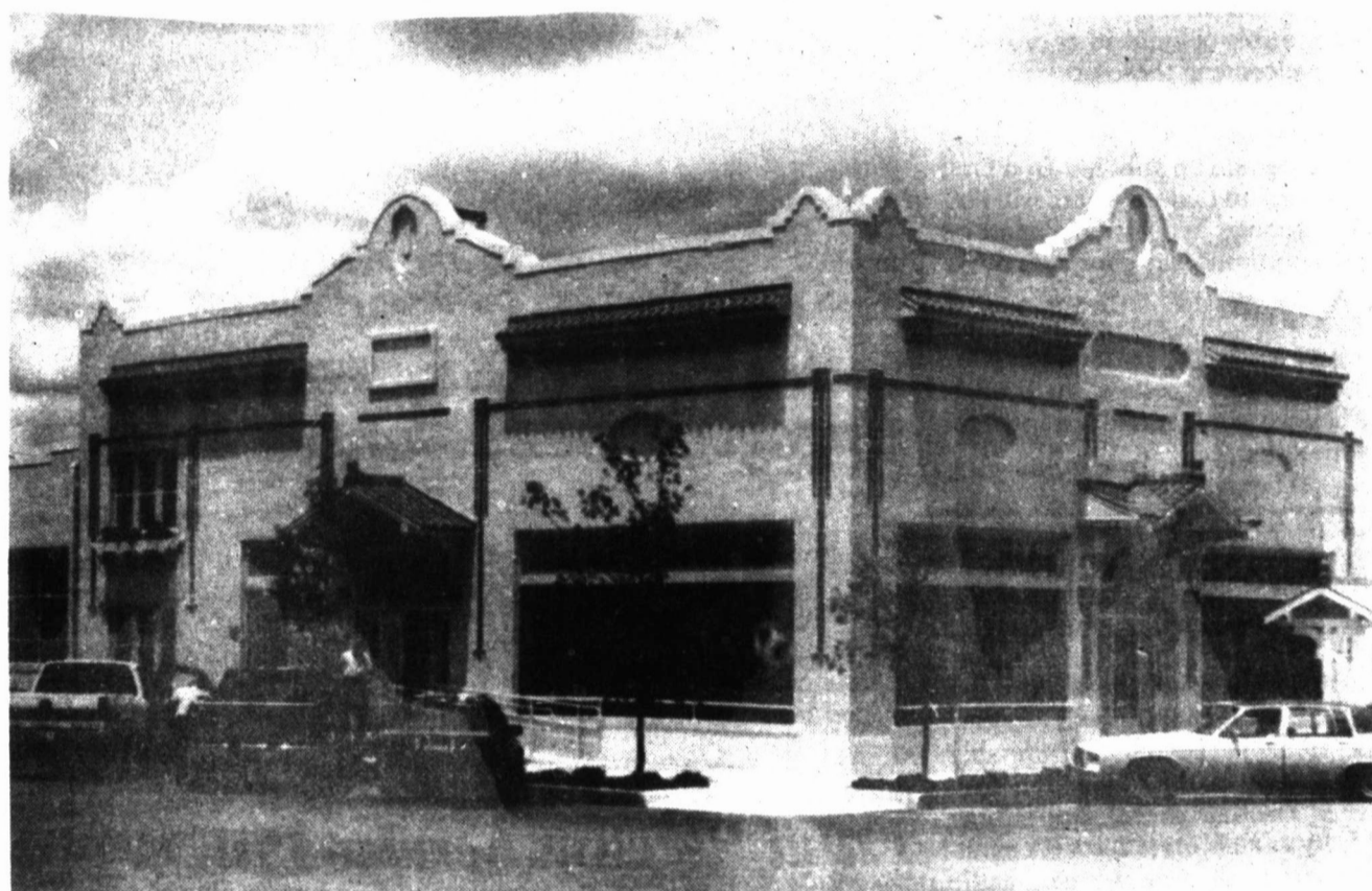
BUILDING RESTORED. Cade Matthews and others have done a beautiful job of restoring the old Alderson Chevrolet Building. The building now sparkles like it did two generations ago when it was new. Fixing up and painting seems to be contagious. A number of other buildings in town are undergoing renovation. Ultimately everyone in the community benefits from such improvements.
