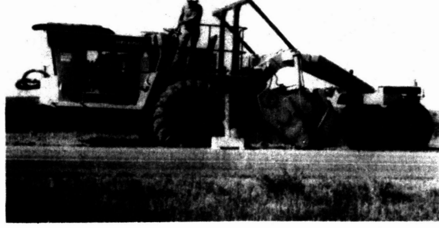
ROAD WORK is continuing on Highway 287 East of Clarendon. The truck at left puts powdered cement on the ground, after which the rototiller-like machine at right incorporates it into the road base. Water trucks then wet down the mixture and big rollers pack the base. Finally, crews spray asphalt to seal the base and top it with hot mix.
