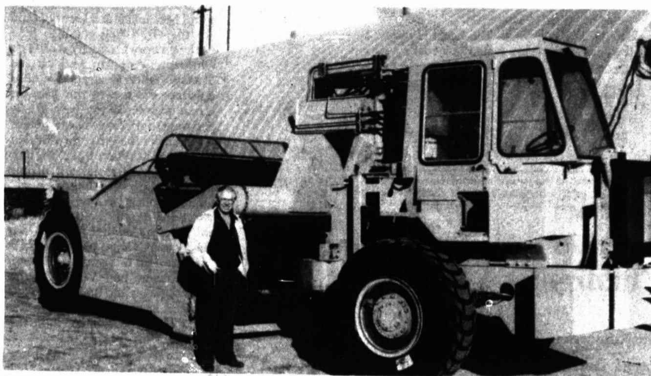
Darrell Leffew and the new CMDCO 252 Scraper.
