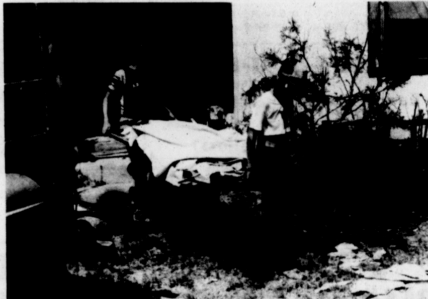
SCOUTS WORK HARD TO SAVE MATERIALS.
