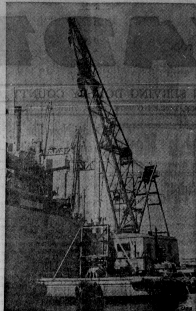
NO SWEAT - The strange looking craft at the Naha Port facilities, Okinawa, is a floating crane. Operated by the 2d Logistical Command, the huge crane is called into action whenever extremely heavy cargo is to be loaded or unloaded aboard vessels. The 100-foot boom has the capability of lifting up to 200,000 pounds and can traverse in a complete circle. The barge has facilities to house and feed its 15-man crew.
