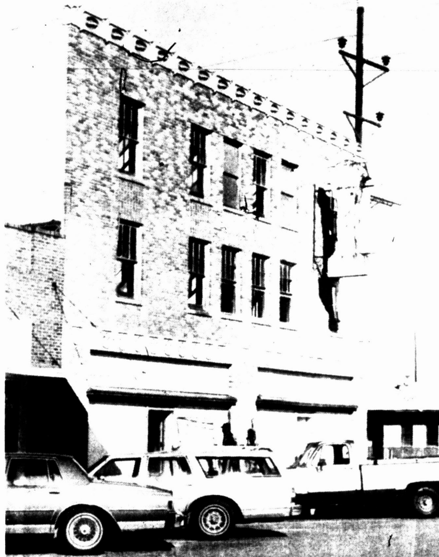
WORKED STARTED ON OLD HOTEL. Workmen began removing trash from the Peabody Hotel on Friday, January 13th.
