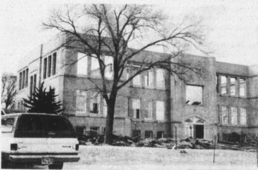
Progress of renovation of the Clarendon High School
